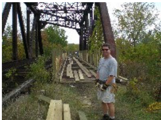
Joe Logan, our civil engineer, gave a hand too.
